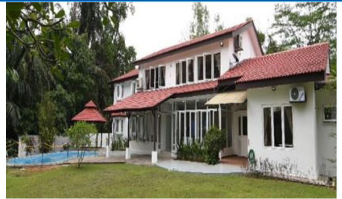
Figure 7: LYC Senior Living, Jalan Gallagher
